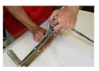
2. Remove vertical hardware from shield using socket wrench, 3/8" socket, and appropriate torx driver.
